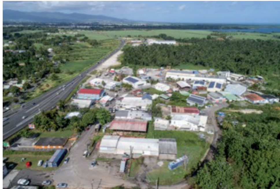
ZAE de Beausoleil, Baie-Mahault
