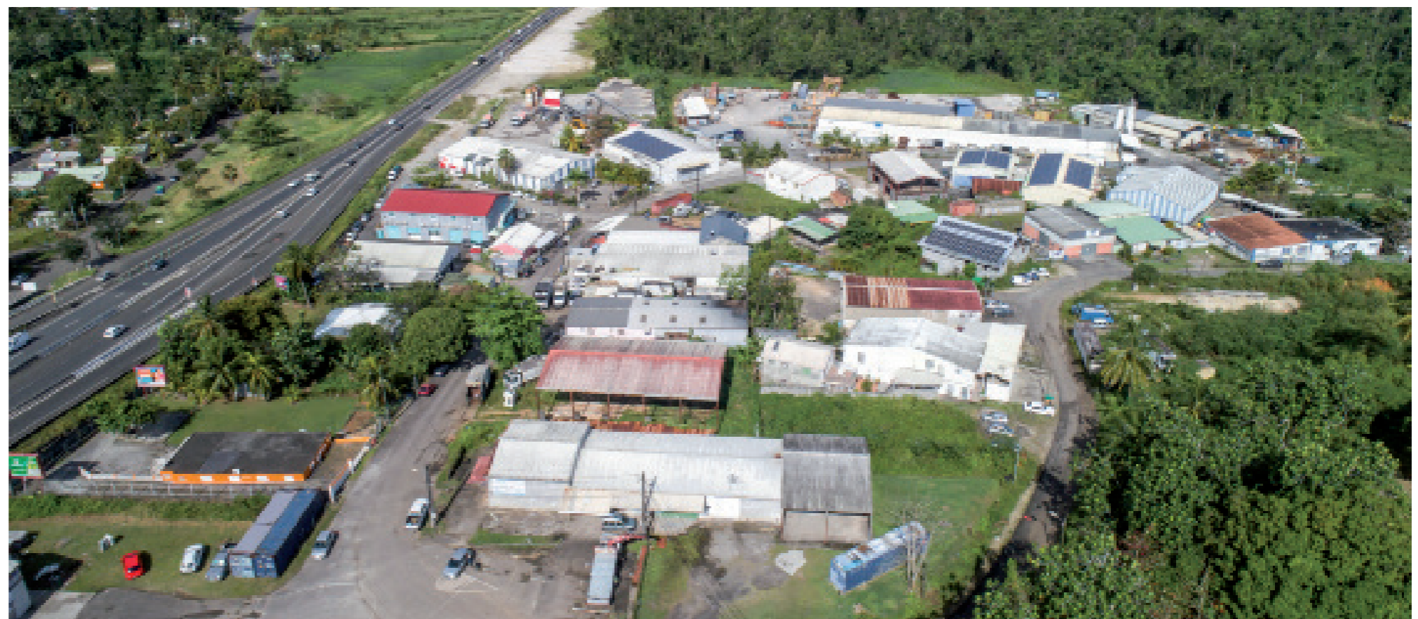
ZAE de Beausoleil, Baie-Mahault
